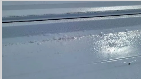
Photo 4: This photo shows blistering, which occurs when there is pressure under the coating.
