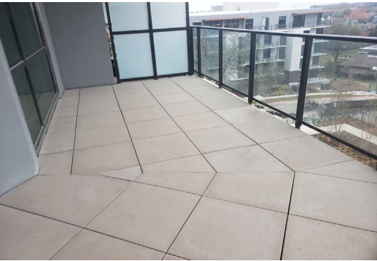
This image was taken after Chamberlin was finished installing the Wausau pedestal pavers.
