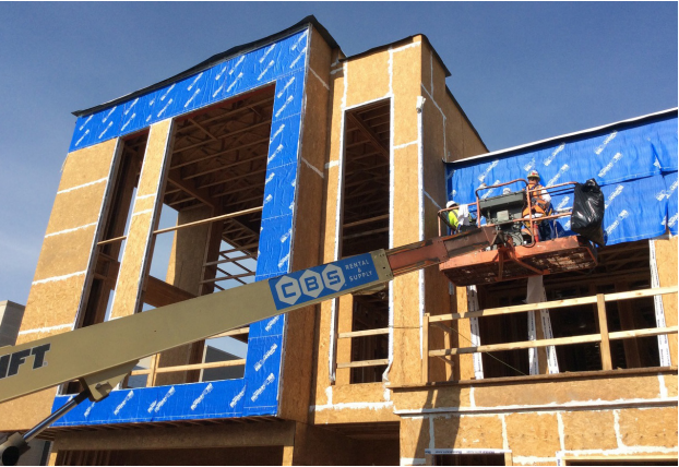
Chamberlin crew working on a weather barrier installation.
