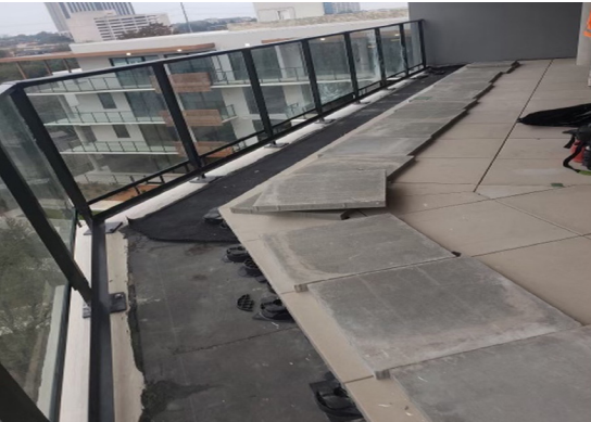
This image was taken during the installation of the Wausau pedestal pavers.
