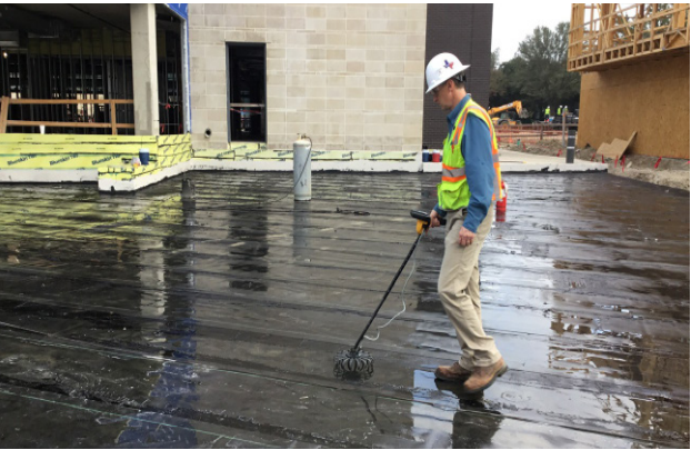
Chamberlin using electric field vector mapping, to help check for waterproofing membrane for breaches.
