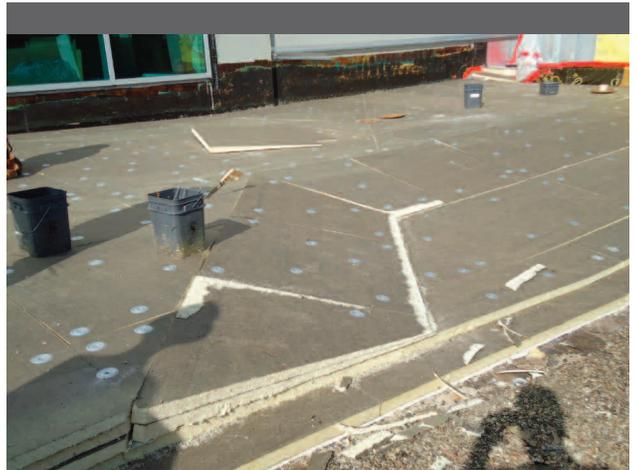
*Insulation was added to the roof area and tapered toward drains.*
