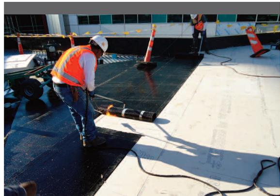
*Chamberlin installed over 10 acres of Soprema's torch-applied roofing system on the terminal.*
