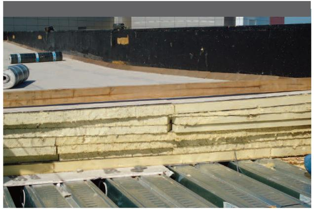
*Chamberlin redesigned the roofing system to allow for proper drainage, adding as much as six inches of extra insulation to meet required slope.*
