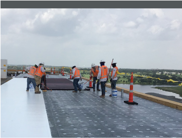
Chamberlin crew members installing membrane over cover board
