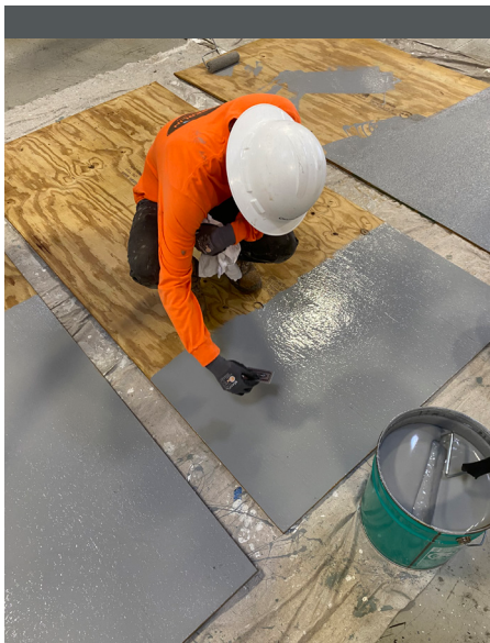
Traffic coating waterproofing apprenticeship
