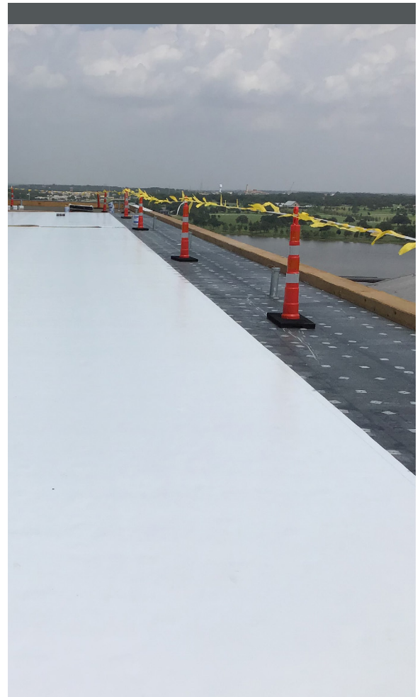
PVC roofing system installation in progress
