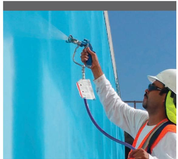
Installing spray-applied air barrier to the exterior wall of The Ford Center.
