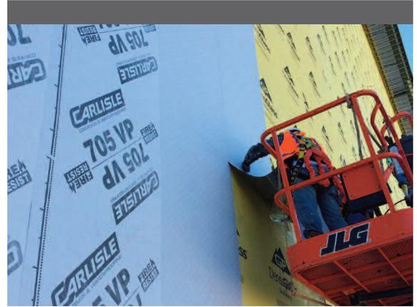
Applying “peel and stick” waterproofing to the north wall of The Ford Center.
