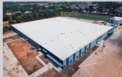
Photo 1: This photo shows a roof that was freshly re-coated.
