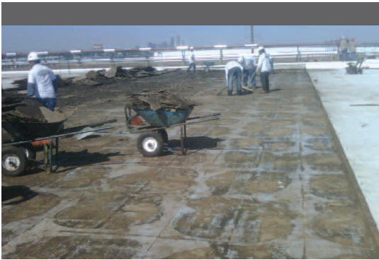
Chamberlin workers removed the existing roof systems.
