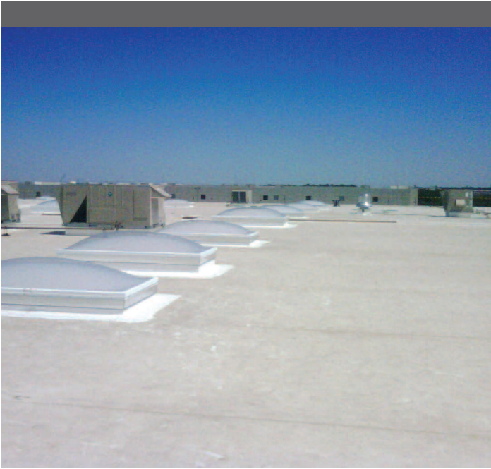
A portion of the completed roof and skylights.
