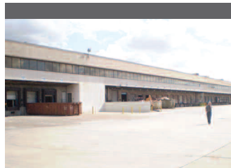
The building's exterior prior to renovation.
