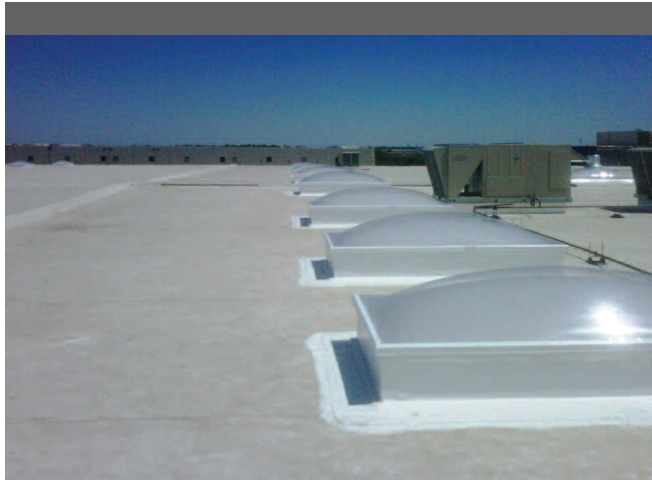
Additional skylights were installed to provide natural sunlight and reduce the need for artificial lighting.
