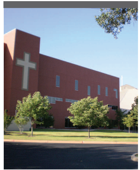
The completed project.
