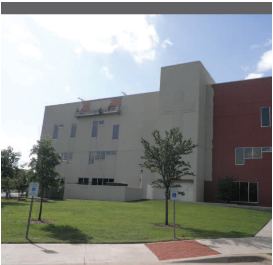
The new elastomeric coating being applied to the church facade.
