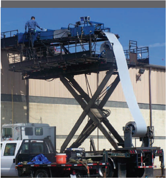
The Archzilla® sheet metal truck custom fabricated material on location.
