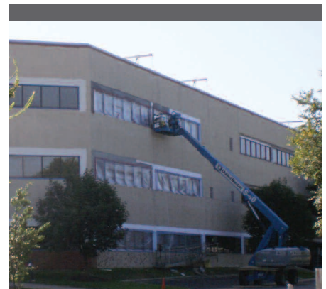
Chamberlin reflashed and recaulked windows.
