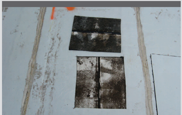
Inspection of the roof system after test failure.
