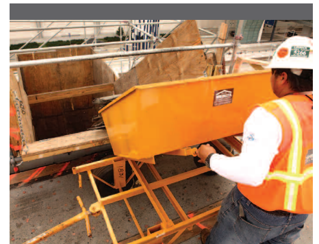
Chamberlin worker unloading debris into the garbage chute.
