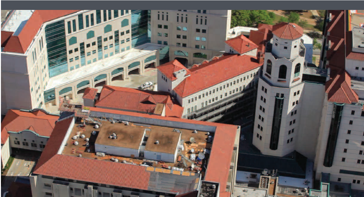
An aerial view of the Memorial Hermann Hospital campus shows the scope of work involved in the emergency repair and roof replacement project.
