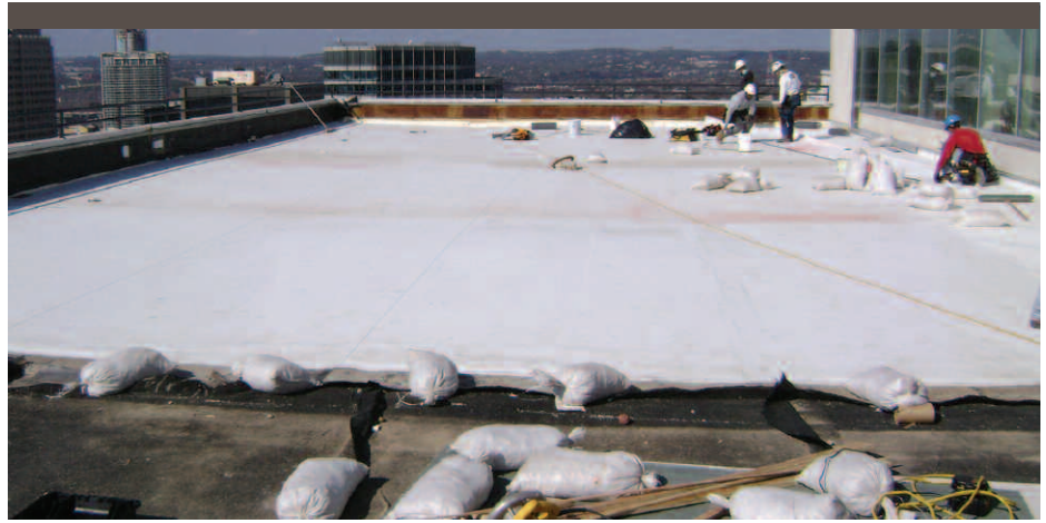
Chamberlin crew installing new, energy efficient TPO roofing system.
