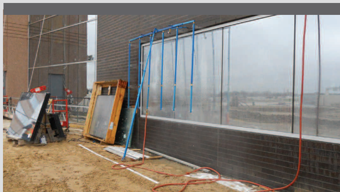
Water penetration testing at a children's hospital annex.
