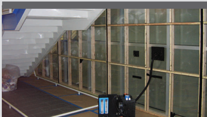
Air infiltration testing at a community college technology center.
