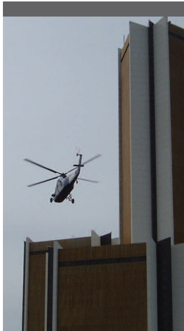
TPO roofing membrane delivered via helicopter
